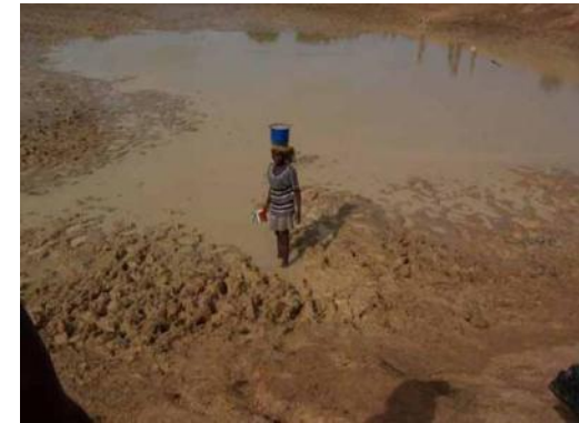
St. Mary's Dam
